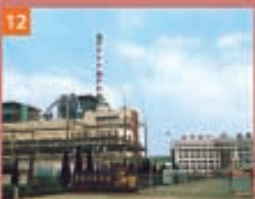
12 Huaiyin Power Plant (1,060MW)
