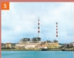
5 Weihai Power Plant (850MW)
