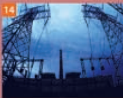
Nanjing Power Plant (640MW)
