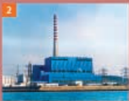
2 Yingkou Power Plant (640MW)
