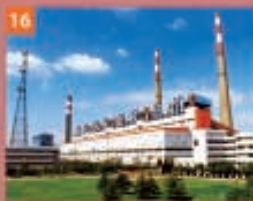
Shanghai Shidongkou First Power Plant (1,200MW)
