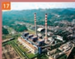
Luohuang Power Plant (1,548MW)
