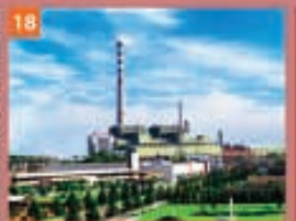
Yueyang Power Plant (725MW)
