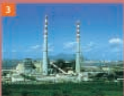
3 Dalian Power Plant (1,400MW)
