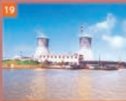
Changxing Power Plant (250MW)
