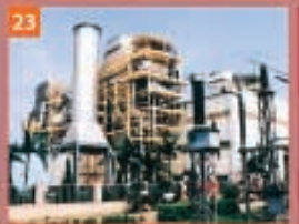
Shantou Combined Cycle Power Plant (103MW)
