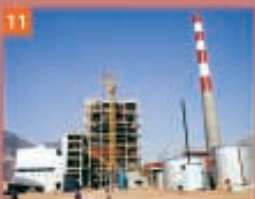
11 Qinbei Power Plant (1,200MW)
