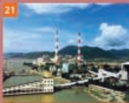
Fuzhou Power Plant (1,400MW)
