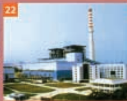
Shantou Coal-fired Power Plant (600MW)
