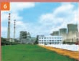
6 Dezhou Power Plant (2,520MW)
