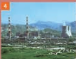
4 Shang'an Power Plant (1,300MW)
