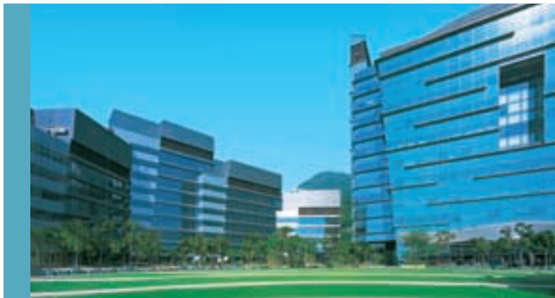
The commercial portion of the Cyberport project was completed on June 28, 2004.
