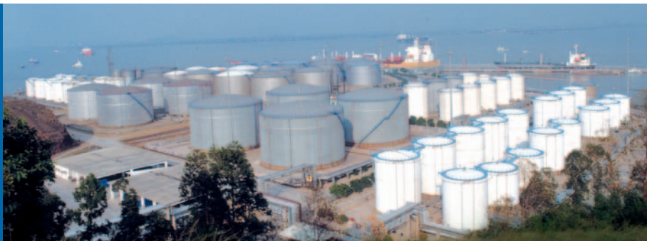
Storage Tank Farm of Xiao Hu Island Terminal
