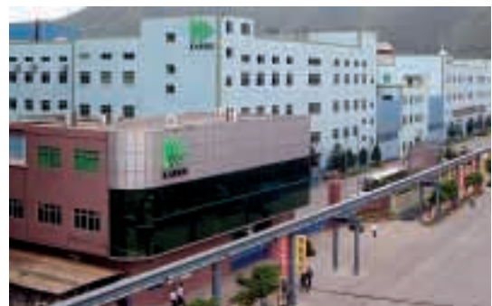
Fenggang Plant 鳳崗廠房
