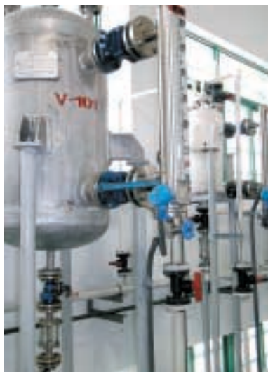
The Chemical Plant in Zhuhai
