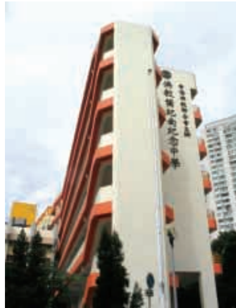
Completed superstructure works for Buddhist Yip Kei Nam Memorial College at Cheung Ching Estate, Tsing Yi Island, New Territories by Chinney Construction Company, Limited
