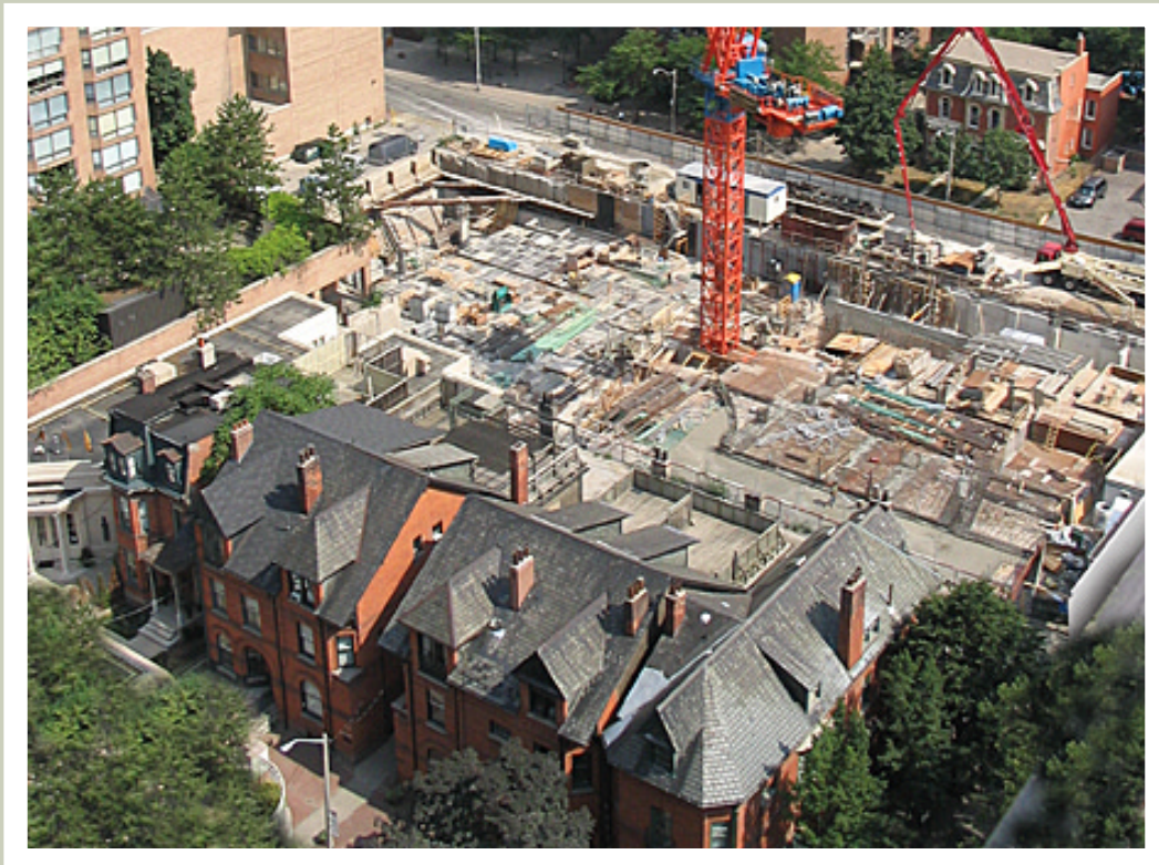
The Group's Canadian project under construction
