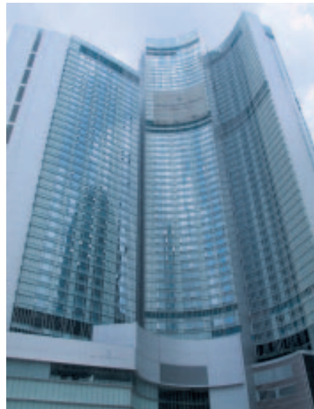
PABX System Solution for six-star hotel — Four Seasons Hotel
