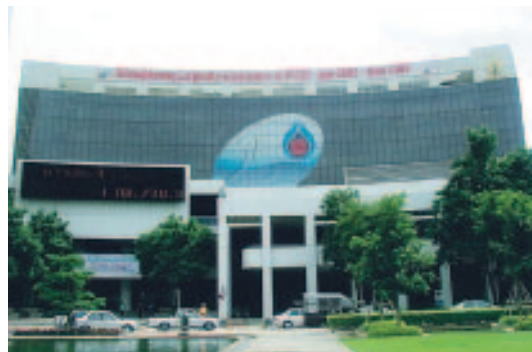
Installation over 1,000 IP endpoints in PTTEP Building — the largest IP Telephony project in Asia Pacific in 2004
