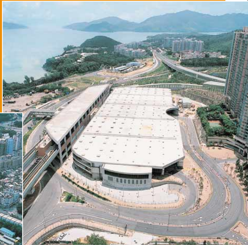
Public Transport Interchange at Wu Kai Sha Station
