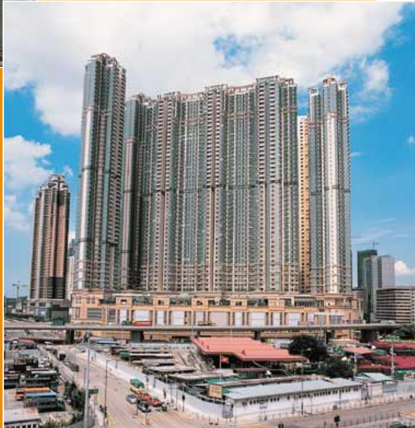
The Pacifica at NKIL 6275 West Kowloon Reclamation
