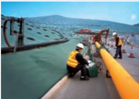
Connection of a pipeline from the North East New Territories landfill site to Tai Po Gas Plant
