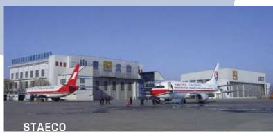
STAECO provides line and base maintenance to Shandong Airlines and specialises in performing heavy maintenance for B737 aircraft for other airlines. Its two hangars can fully dock five B737 aircraft.
