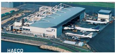
HAECO provides line maintenance for about 70 airlines at Hong Kong International Airport. It also performs heavy maintenance in a hangar which holds three wide-bodied aircraft fully docked with an additional two nose-in. Its second hangar will open at the end of 2006 and have capacity for two B747 and one aircraft of up to B787 size fully docked.
