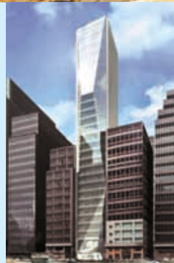
From top: Liu Chong Hing Bank Building on site construction status; Prospective view
