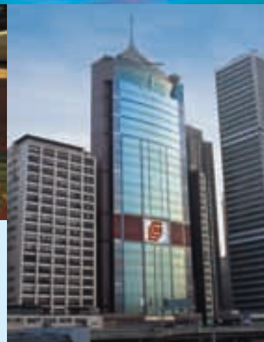
Western Harbour Centre: Grand lobby and external view
