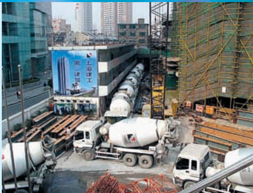
Shanghai LCH Centre, on site construction status
