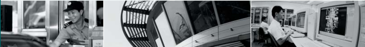
Eastern Harbour Crossing – one of the three cross harbour tunnels in Hong Kong.
