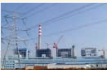
Wushashan Power Project
