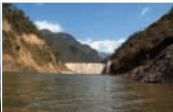
Lixianjiang Hydropower Company
