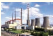
Zhang Jia Kou Power Plant
