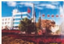
Dou He Power Plant
