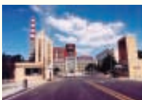
Gao Jing Thermal Power Plant
