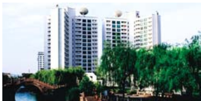
Suzhou Garden Villa high rise apartments 錦華苑多層公寓樓
