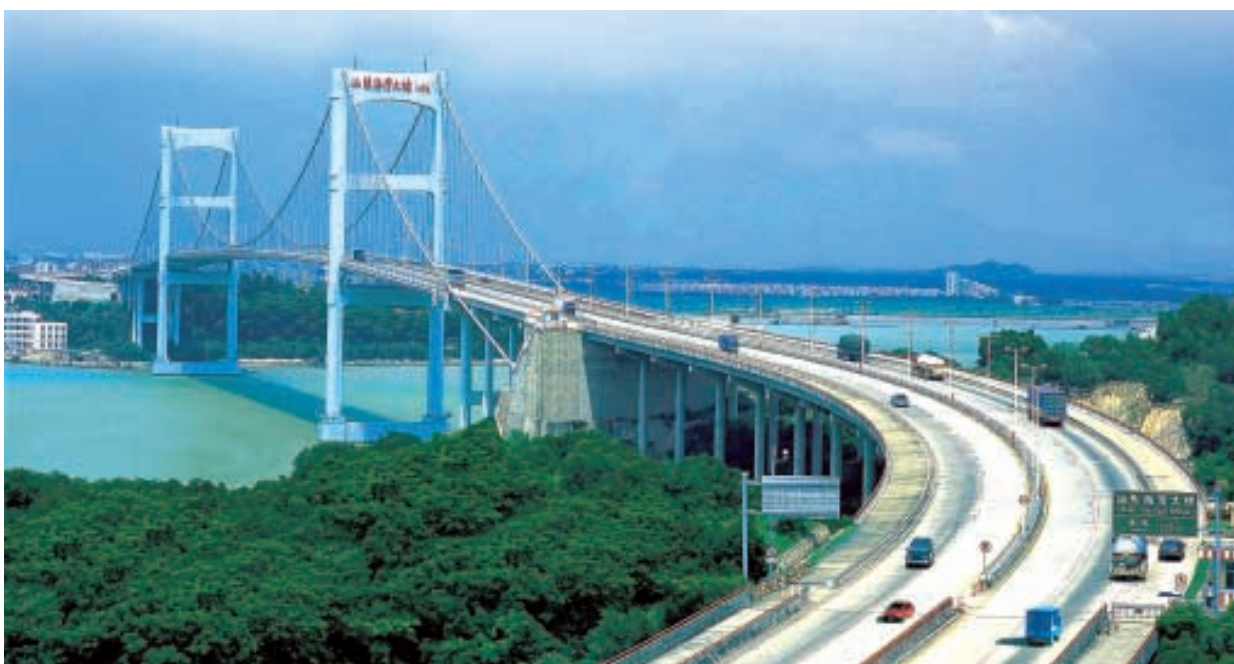
Shantou Bay Bridge
