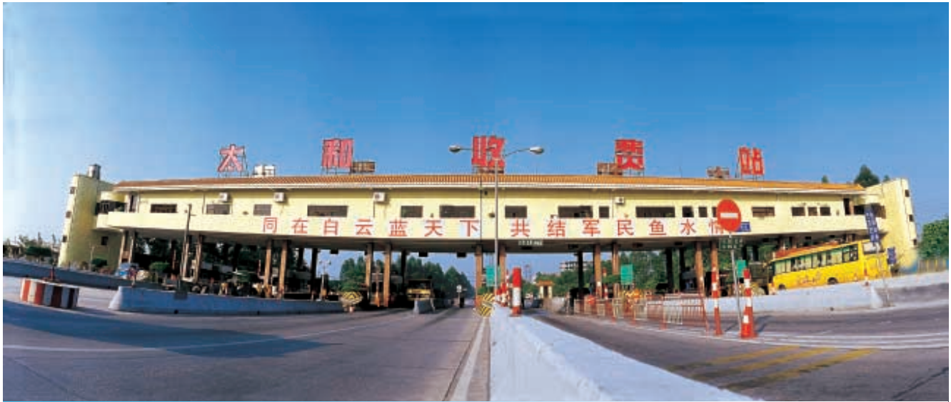
Taihe Toll Station
