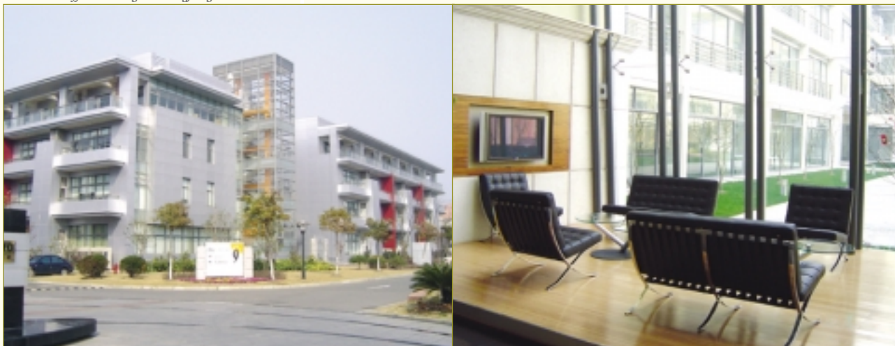
Intellectual Office Buildings at Zhangjiang Micro-electronics Port 張江微電子港智能化辦公大樓
