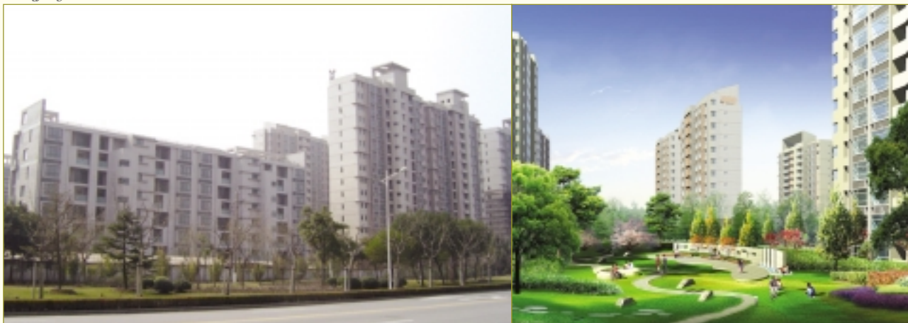
Zhangjiang Tomson Garden (Phase 2)(under construction) 張江湯臣豪園二期(在建中)
