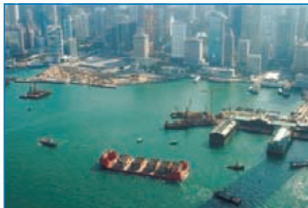
Central Reclamation Phase 3
