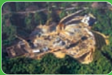
Sha Tin Heights Tunnel and Approaches
