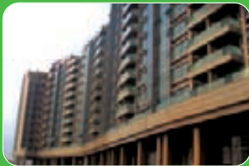
New Kowloon Inland Lot 6196, Cornwall Street, Superstructure
