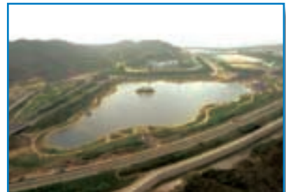
Infrastructure for Penny's Bay Development-Contract 1
