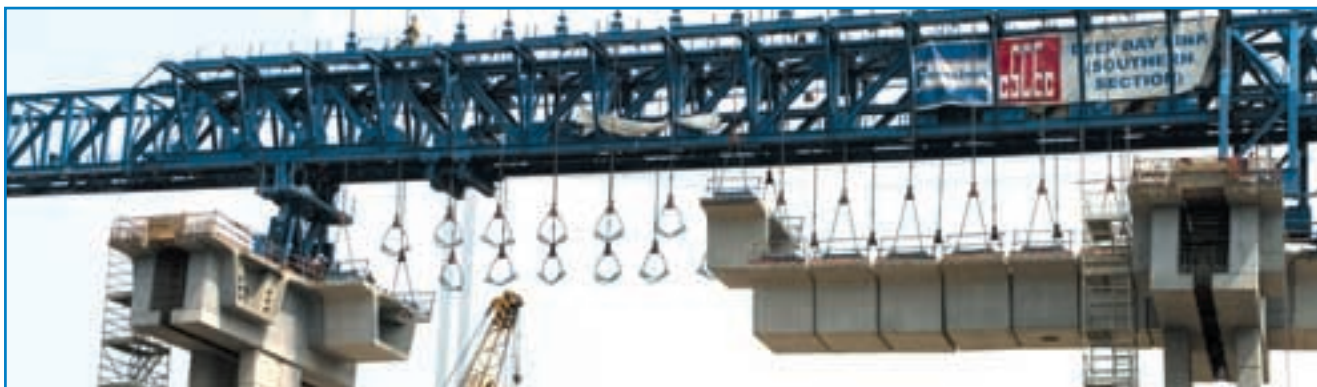
Pre-cast structures are related to the construction business of the Group.
