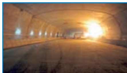
Sha Tin Heights Tunnel and Approaches
