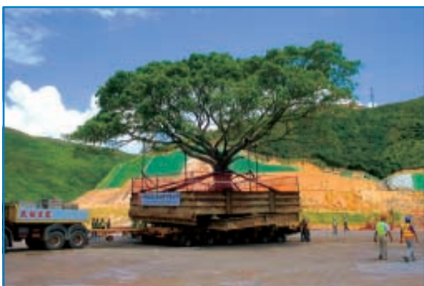
Trees conservation is also of high importance to environmental conservation. During the construction period, the Company built safety fencing around big trees for protection.
