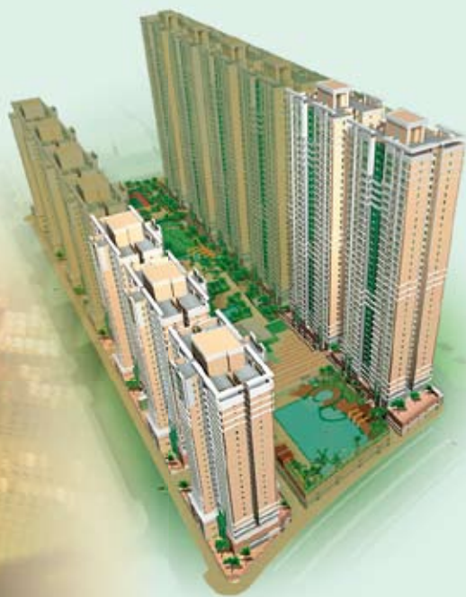
Stage 1 of Nova City was launched to a strong market reception. Superstructure works for Stage 2 was commenced in October.
