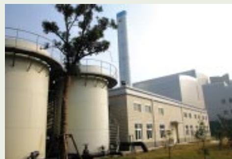
The Group has also entered into the business of complete solid waste incineration systems through participating in a solid waste incineration BOT project.
