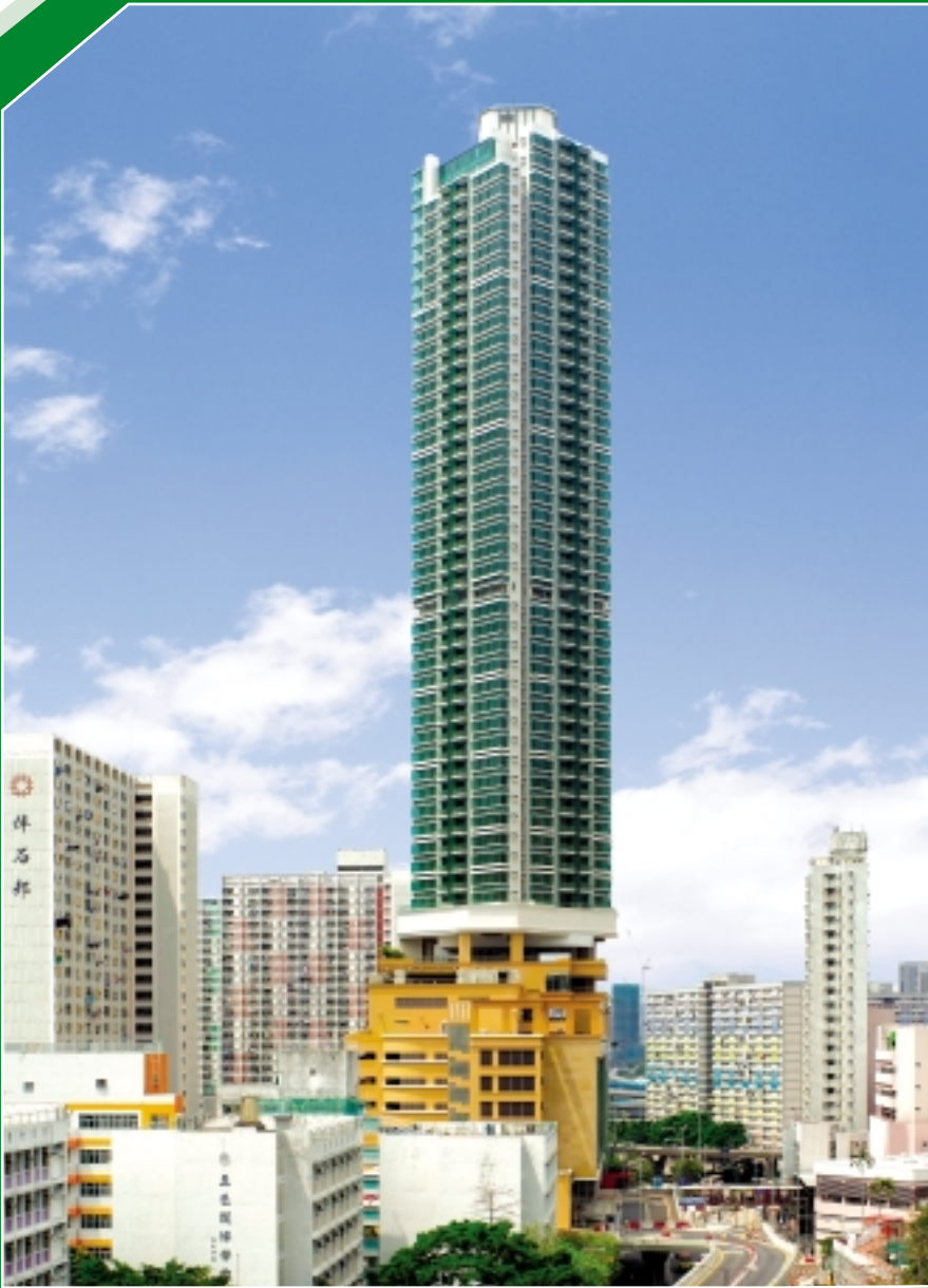
No. 8 Clear Water Bay Road Development above Choi Hung MTR Station
