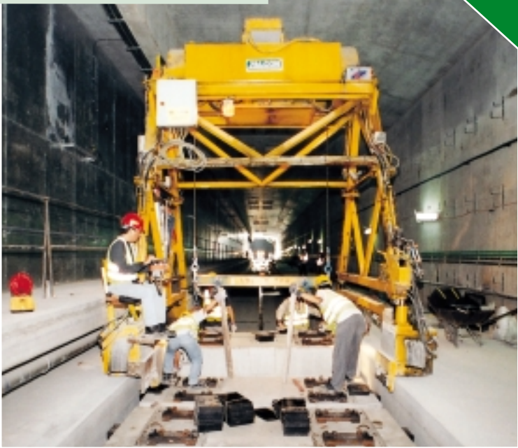
KCRC East Rail Extensions - Permanent Way for Lok Ma Chau
