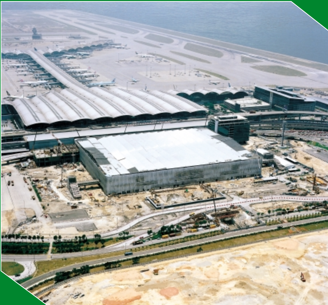
SkyPlaza and Associated Works at Hong Kong International Airport
