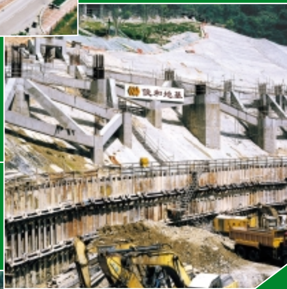
Site Formation and Foundation Works for School at Shum Wan Road
