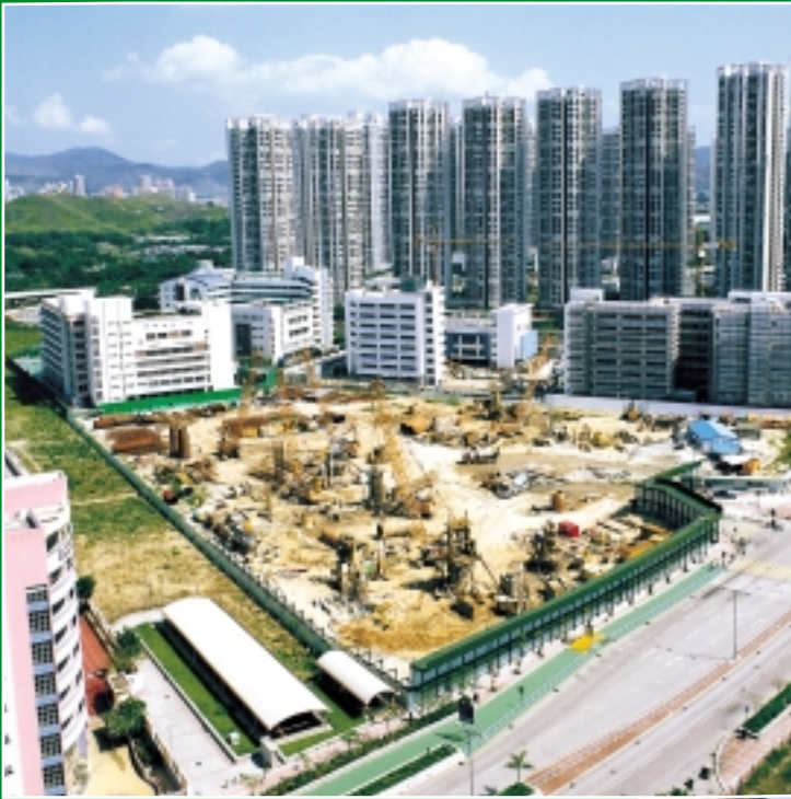
Foundation for Tin Shui Wai Area 104
