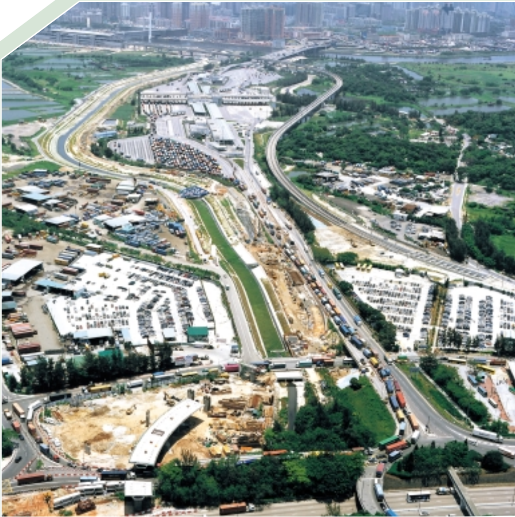
Improvements to San Tin Interchange
