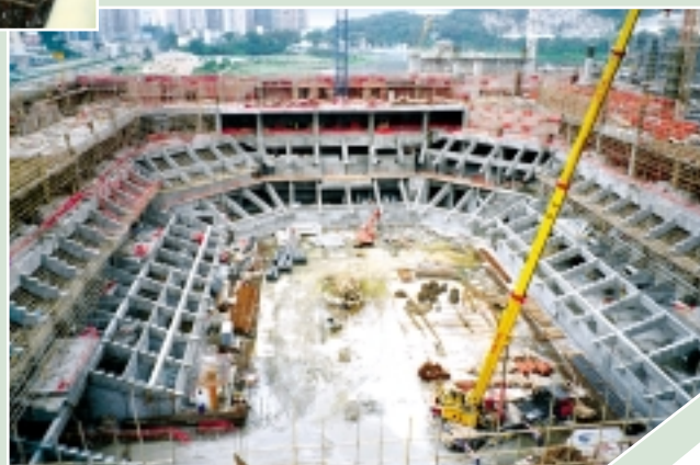
Event Centre Superstructure Construction at the Venetian, Macau
