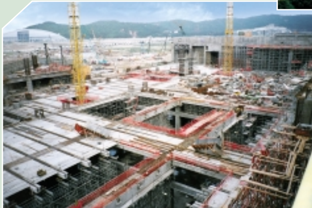
Congress Centre Superstructure Construction at the Venetian, Macau
