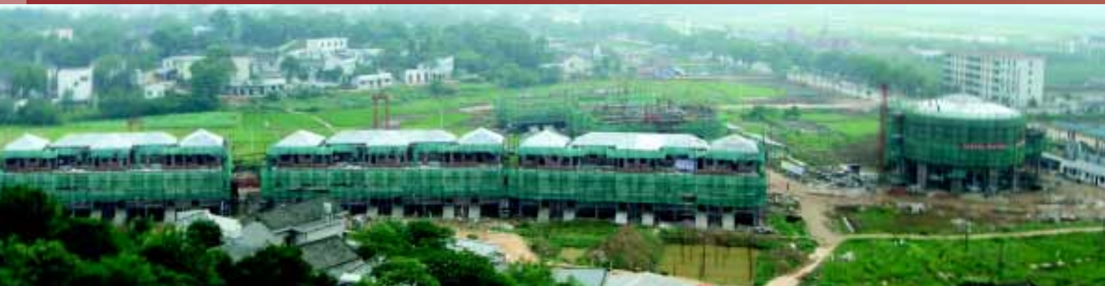
Phase I of Beverly Hills, Changsha (under construction)
