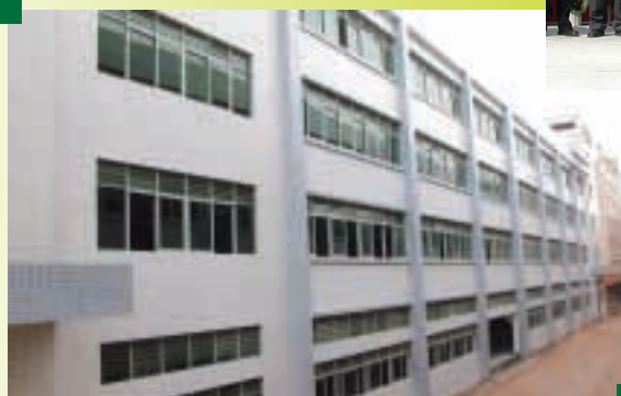
Changing new factory
