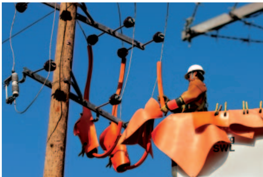
Overhead line training
