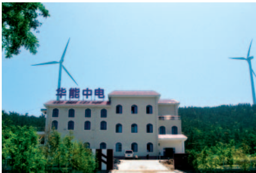
Changdao Wind Farm, Shandong Province
