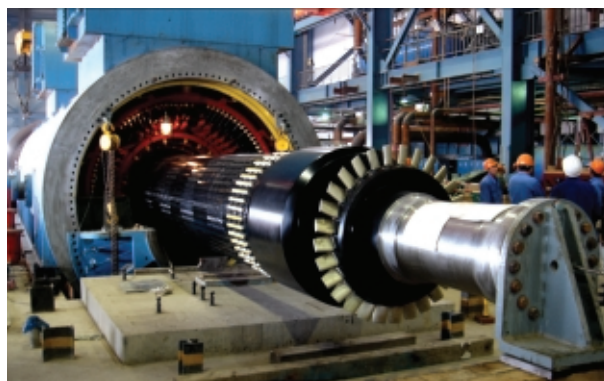
Installation of power generation at Huanghua Power Plant
