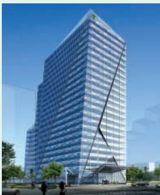
Designed by Tange Associates of Japan, this signature integrated office and retail development will be an impressive addition to the Shanghai skyline.
