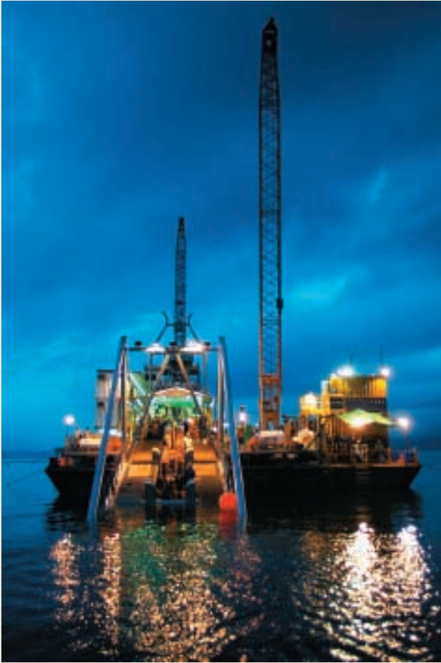
Submarine pipes have been laid in preparation for the delivery of natural gas from Guangdong LNG terminal to Hong Kong and China Gas Production Plant in Tai Po.
