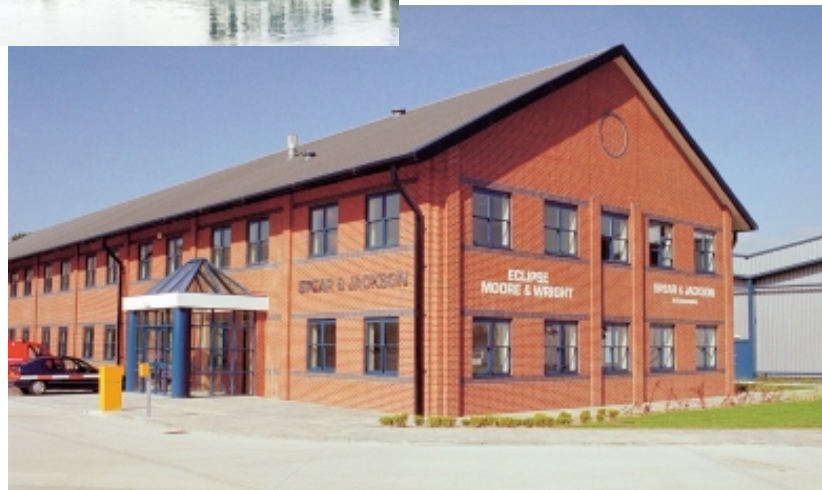
Office and Plant Sheffield, United Kingdom
