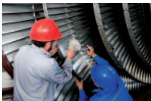
→ (Left) Construction work at Fangchenggang → (Right) Turbine blade cleaning at Fangchenggang
