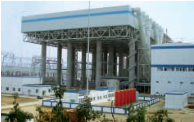
Air-cooling facility of Jinjie Energy
