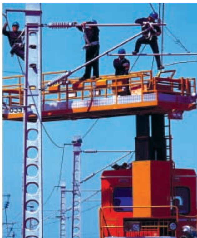
Maintenance of electric railway
