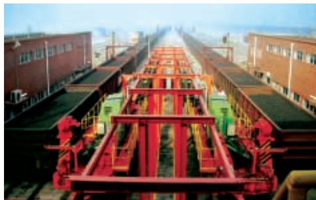
Port-entry line of Huangwan Railway
