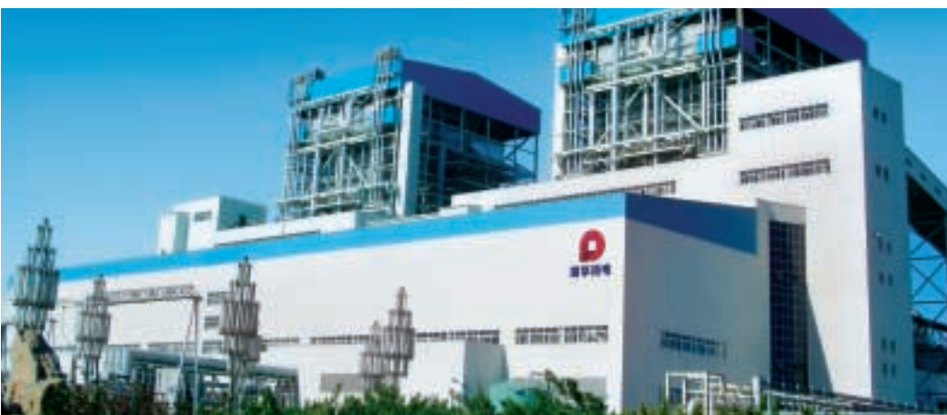
Generation units at Phase I of Huanghua Power
