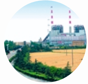
Pingwei Power Plant
