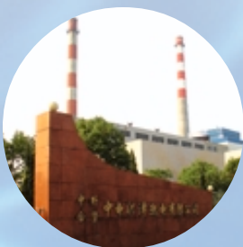
Hongze Power Plant
