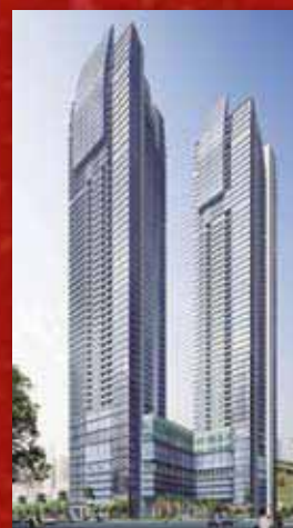
THE ST. FRANCIS TOWERS* MANILA, THE PHILIPPINES
