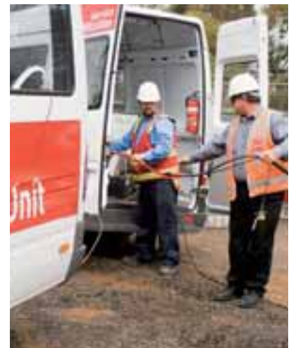
CitiPower's network covers 157 square kilometres, encompassing Melbourne's central business district and inner suburbs.
