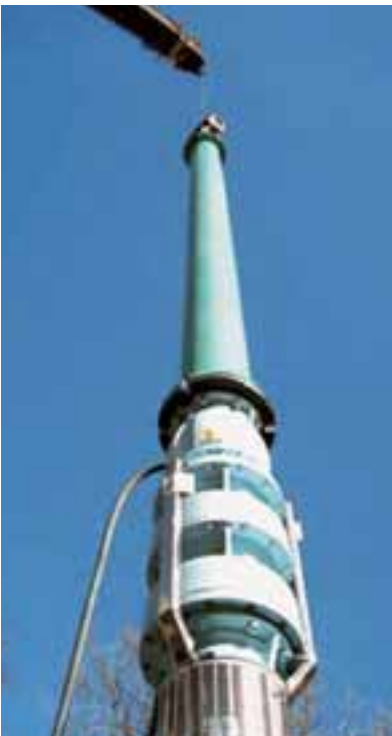
Cambridge Water supplies fresh water to customers in South Cambridgeshire, the United Kingdom.
