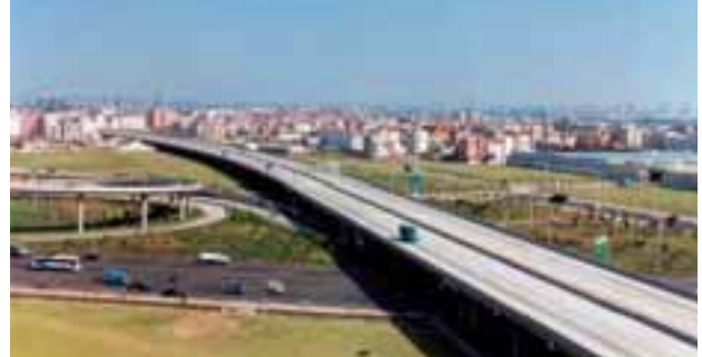
The Guangzhou East-South-West Ring Road achieved a satisfactory performance, with increases in traffic flow and toll revenue.
