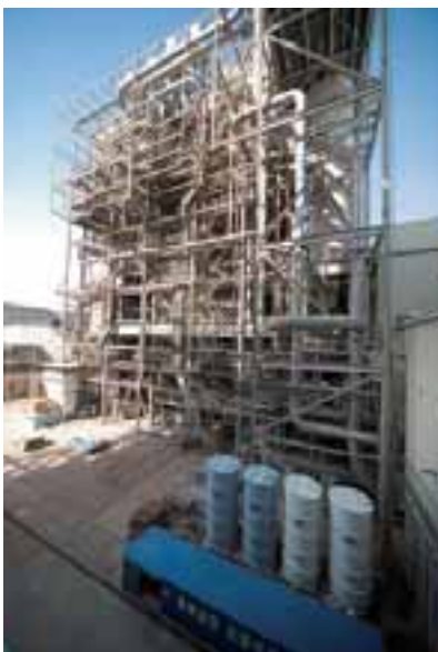
The Zhuhai Power Plant continues to be one of the most efficient, reliable and safe plants in Mainland China.
