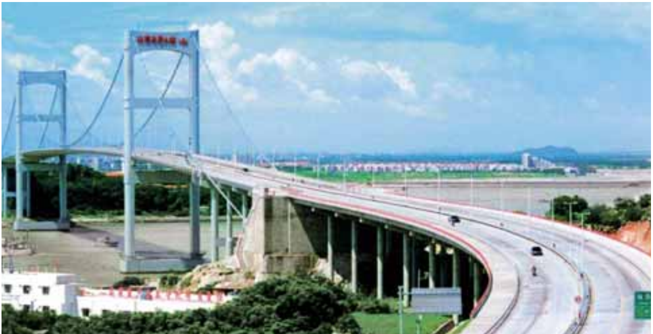
The Shantou Bay Bridge achieved double-digit growth in toll revenue during the year under review.
