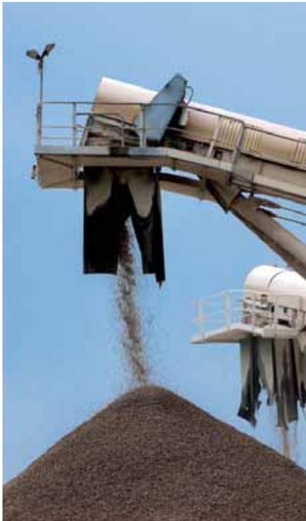
Alliance is the market leader in the territory's concrete and aggregates industries.
