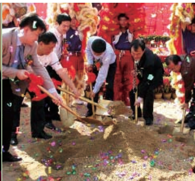
The Group acquired premium land parcels for sustainable growth. Ceremony on commencement of construction work for Fairyland Phase II in Zhongshan City.
