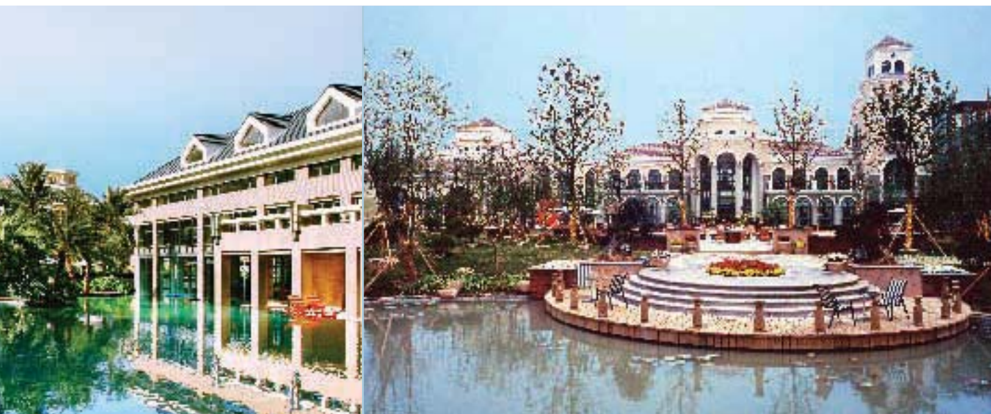
Lakeside Palace project is located on shore of Jinjihu Lake in Suzhou Industrial Park. Its prime location and plentiful scenic resources are focus of the market.
