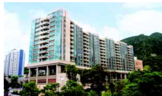
New Kowloon Inland Lot 6196, Cornwall Street, Superstructure
