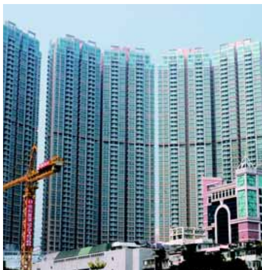
TWT 398, Tai Ho Road, Tsuen Wan, Superstructure
