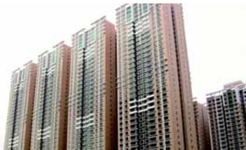
Construction of Nova TaiPa Gardens, Phase 2B
