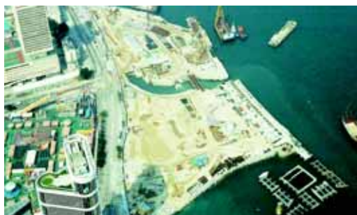
Central Reclamation Phase 3
