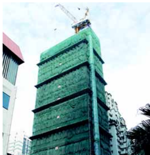
Main Contract for Proposed Commercial Building at 196-206 Queen's Road East
