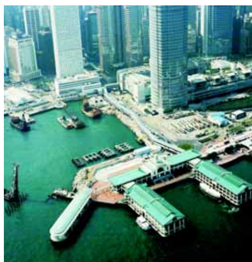
Central Reclamation Phase 3
