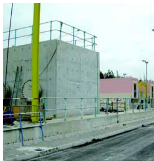
Upgrading of Siu Ho Wan Sewage Treatment Plant – UV Disinfection Works
