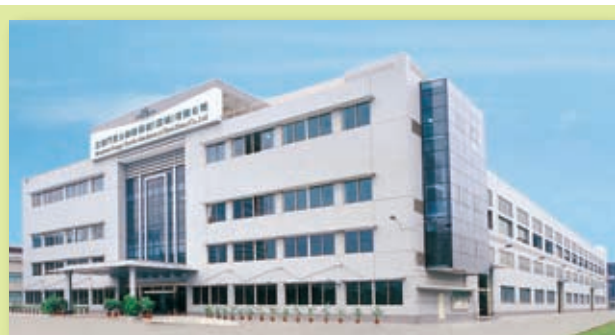
Monforts Fong's Manufacturing Plant
