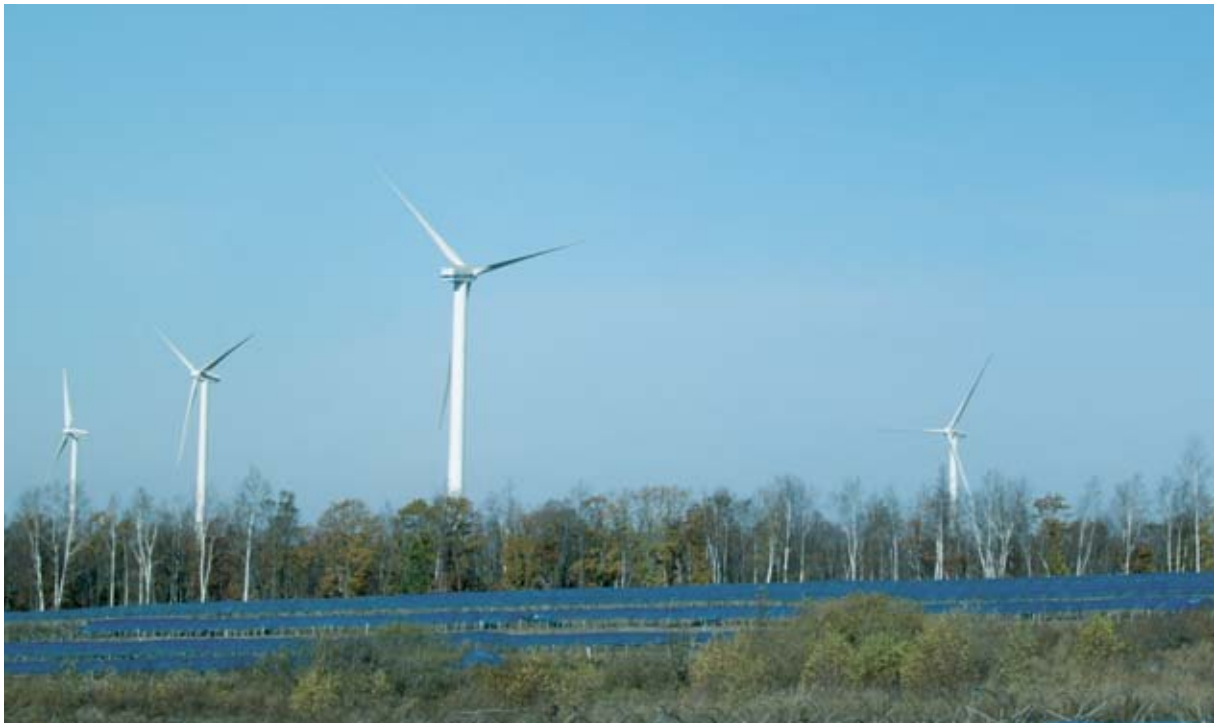
Wind-powered Station, Heilongjiang 黑龍江風力發電廠
