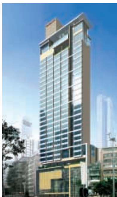
Leighton Road project
