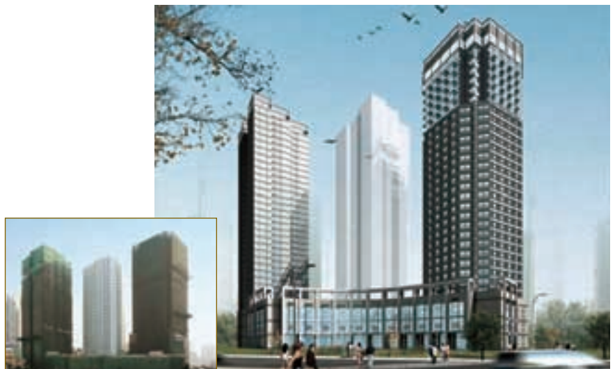
Distressed property project in Qingdao - before and after
