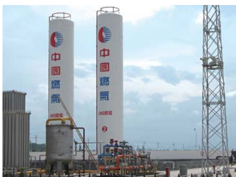
Left: Construction site of mid-range pressure natural gas network in Wuhu Right: Liquefied Natural Gas (LNG) tanks
