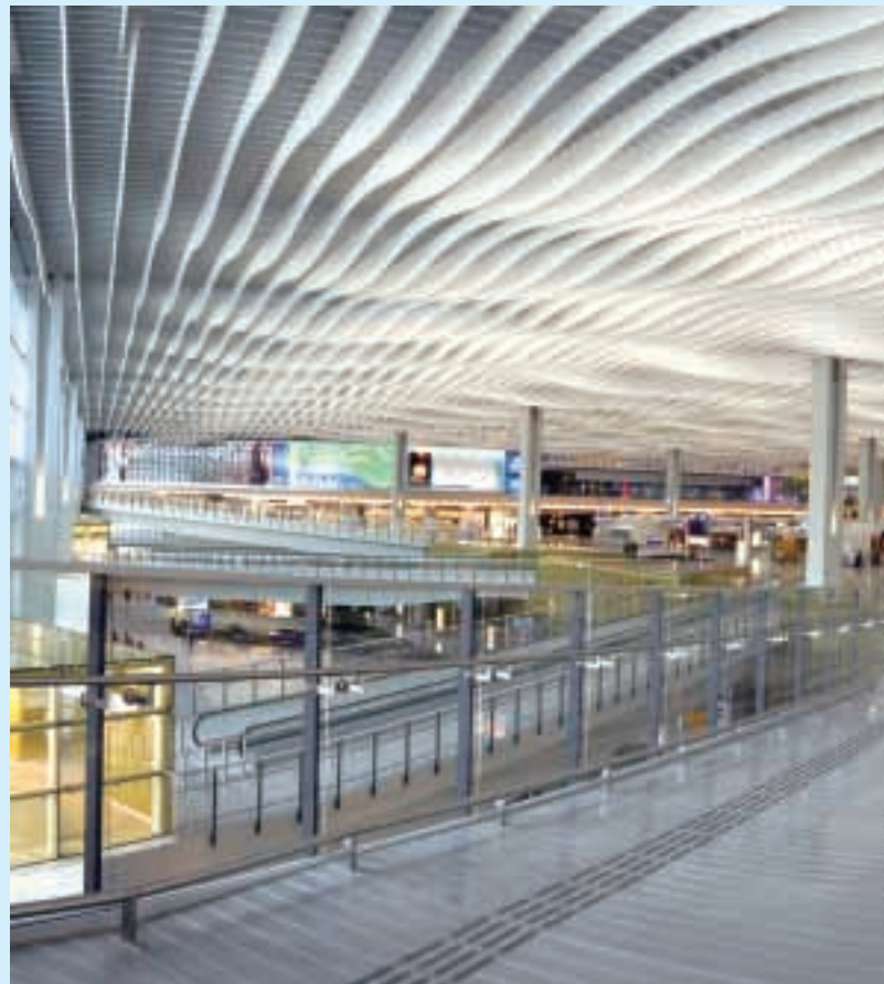
(left and bottom) Hong Kong International Airport SkyPlaza and related civil engineering works
