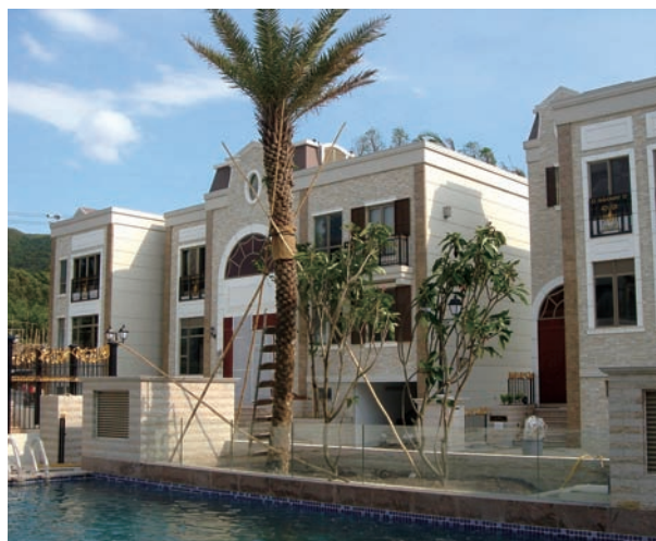
Construction work for the residential development at 1 Fairview Park Boulevard of Yuen Long, New Territories undertaken by Chinney Construction Company, Limited
